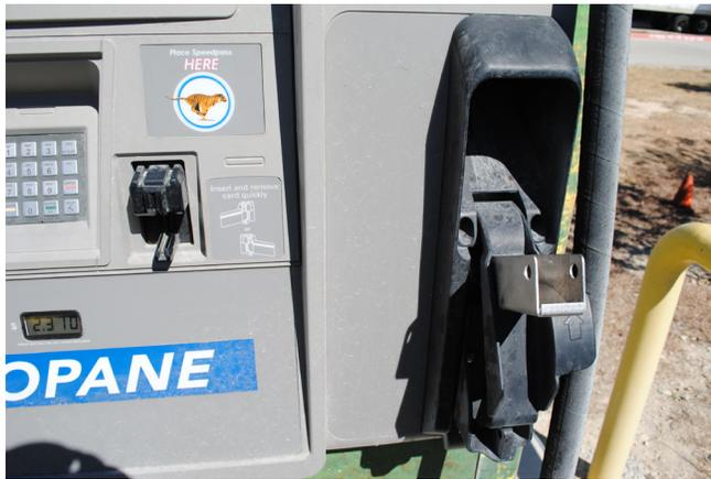
Figure 19. Self-Service Hose-End Valve Interlock Switch
