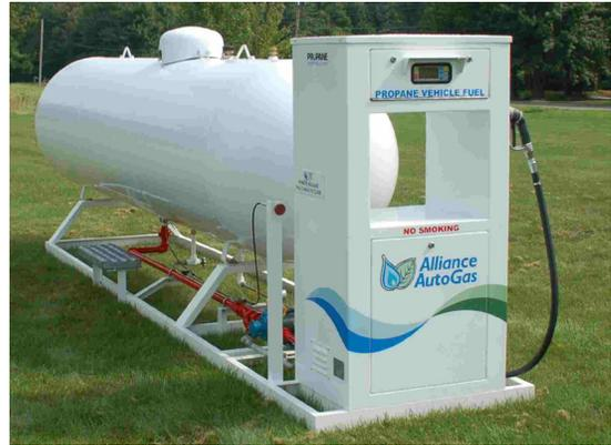
Figure 17. Horizontal Tank Skid and Dispenser Meter/Control Unit
