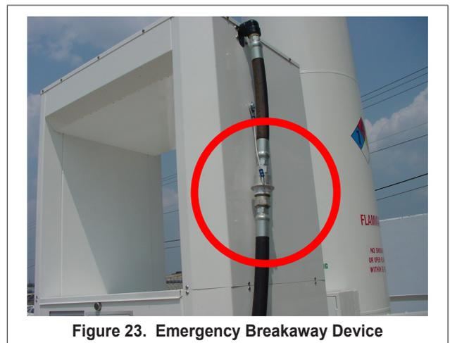
Figure 23. Emergency Breakaway Device
