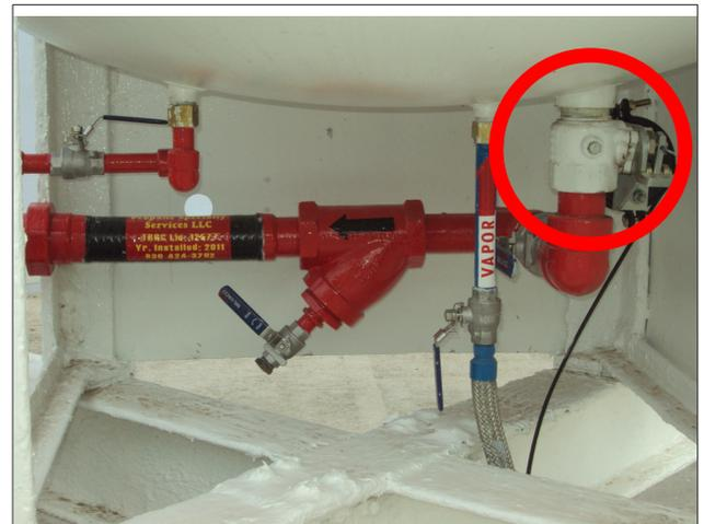
Figure 25. Internal Valve With Automatic Shutoff
